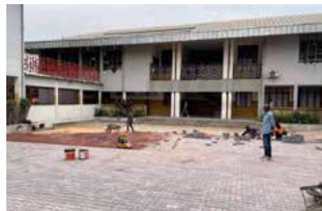
New UPC Clinic/Hospital under construction
